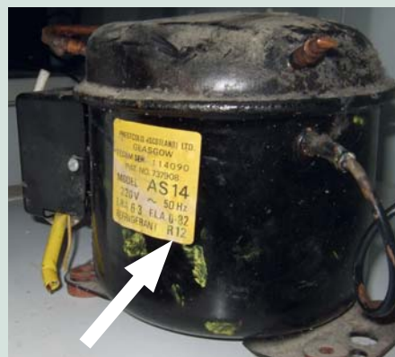
Fridge compressor marked with R12
